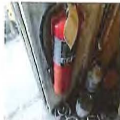
hang new extinguisher on wall
